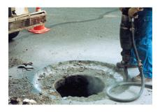
Break and cut 10cm around the manhole at a 90 degrees angle
