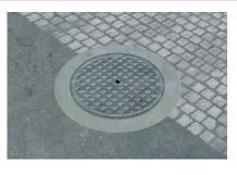
The final aspect of the manhole is important and it should be integrated in the road design
