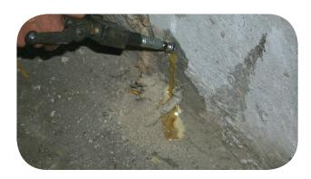
Drill a hole in the concrete at 45 degree angle in order to intersect the crack or the leaking construction joint.
